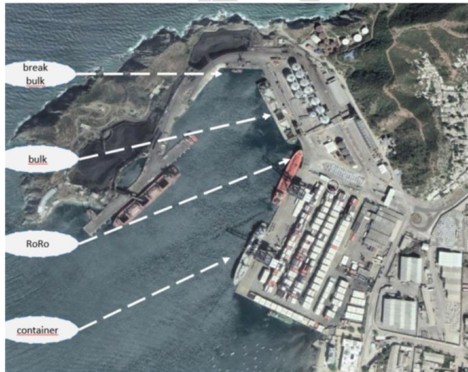
Exhibit 81 Aerial Image of Port of Santa Marta
